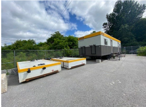
Office trailer with water & septic holding tanks
