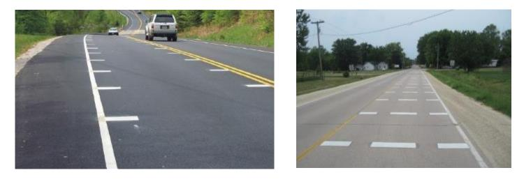
What It Is: Peripheral transverse bars are a series of pavement markings along the edge of the travelled lane widths. The series of markings is placed progressively closer together with distance.
