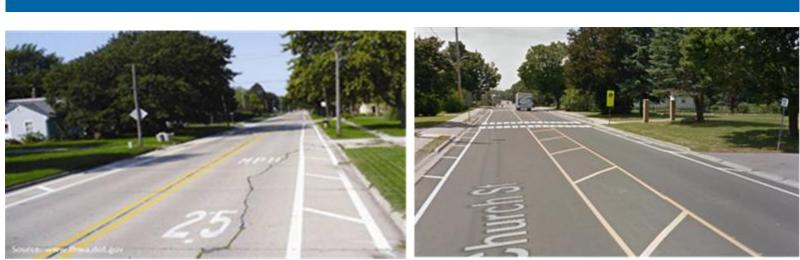
What It Is: Reducing lane widths using pavement markings or other features (for example bicycle lanes or pavement texture).
