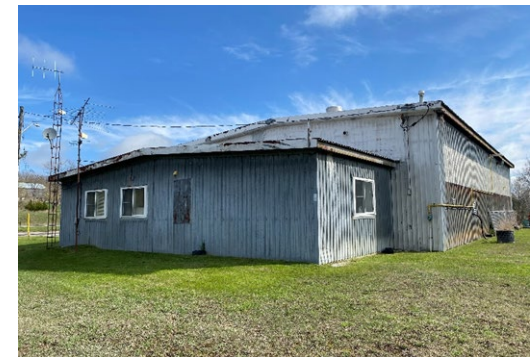
Condition of aging facilities
