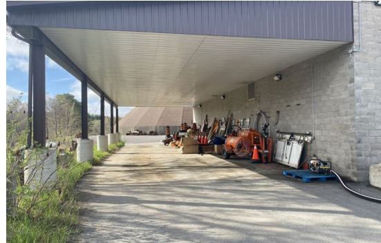
Equipment stored outside
